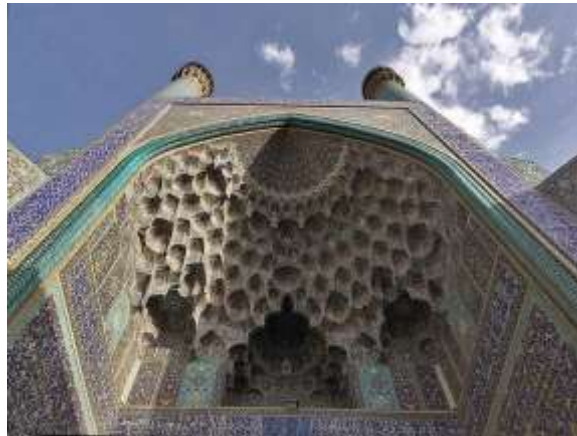
Image 13- The muqarnas decoration of the entrance way of Imam Mosque of Isfahan ( www.eadabt.ir )
